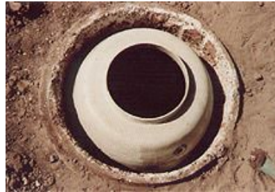
◀A liner inserted into an existing manhole.
