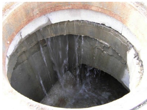
A typical deteriorated manhole showing infiltration. (picture courtesy of waternetsurvey.com )
