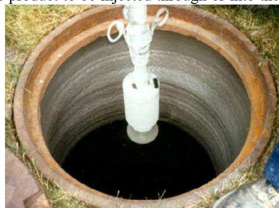
Spray lining of a manhole with a specially designed spray nozzle. Picture courtesy of AP/M Permaform.
