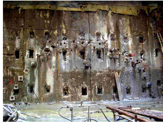
An arch of borehole installed using HDD technology as part of a ground stabilisation programme prior to a major tunnel installation.
