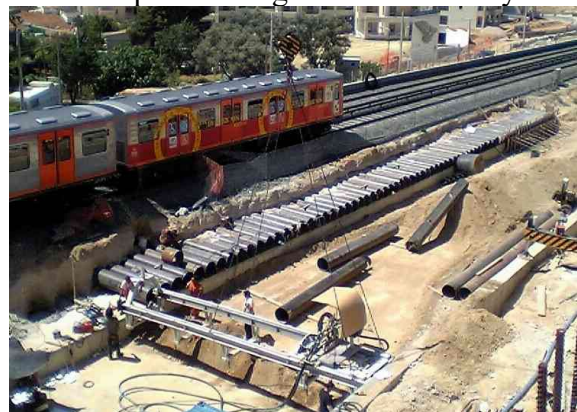
A line of pipes installed using pilot auger microtunnelling technology as the roof section of a pipe arch for an under-rail tunnel installation.
