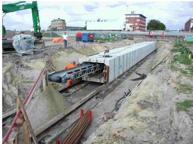
Installing a box section under a railway embankment. In this instance using pulling rods to apply the 'jacking' force as opposed to rear positioned hydraulic jacks. Picture courtesy of HMS Machines BV.
