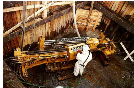
Using HDD to install ground remediation drainage pipelines. Note the personnel protection used for the crew. Picture courtesy of Mining Communications Ltd.
