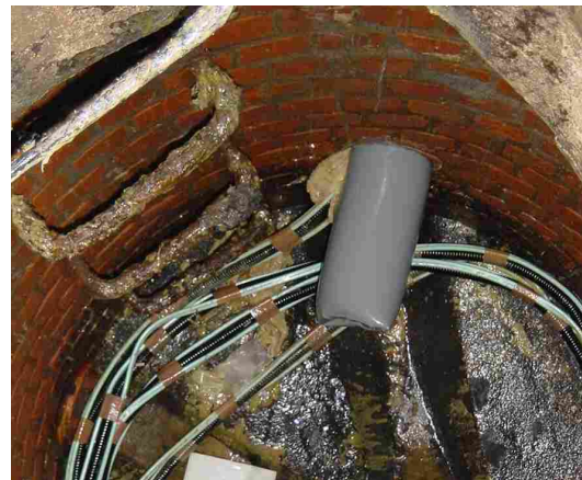
'Inversion Lining' technology being used to install fibre optic cabling in a lateral sewer connection for a residential or business feed. Picture courtesy of Epros GmbH.
