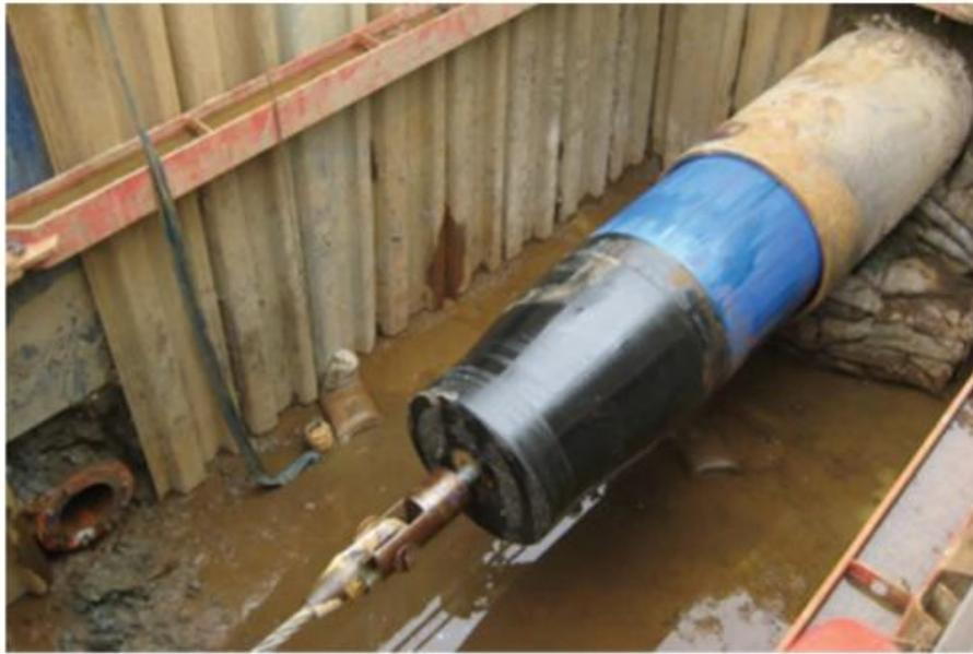
**Figure 3. Die drawing a 1030mm SDR 51 pipe on the Vyrnwy aqueduct, United Utilities.**
