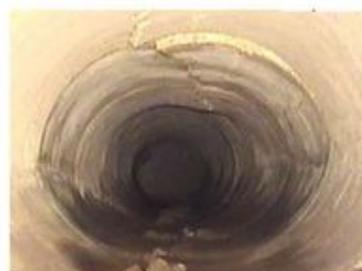
Figure 3: Host pipe condition III [DWA-A 143-2].
