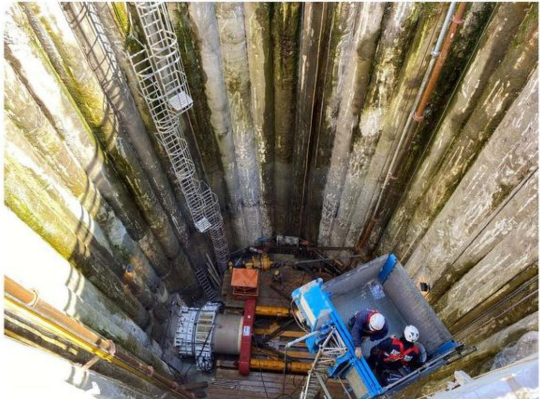
Figure 12. Jacking process, from top left: pit 2, intermediate jacking station, pit 3 (bottom)
