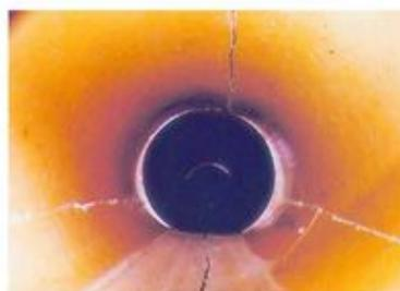
Figure 2: Host pipe condition II [DWA-A 143-2].
