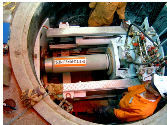
Pilot auger boring is used to install a new lateral connection pipeline.
