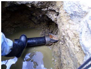
A small footprint pipe bursting system (right) being utilised to replace a deteriorated PVC lateral pipe (left).
