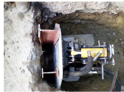
A small footprint pipe bursting system (right) being utilised to replace a deteriorated PVC lateral pipe (left).
