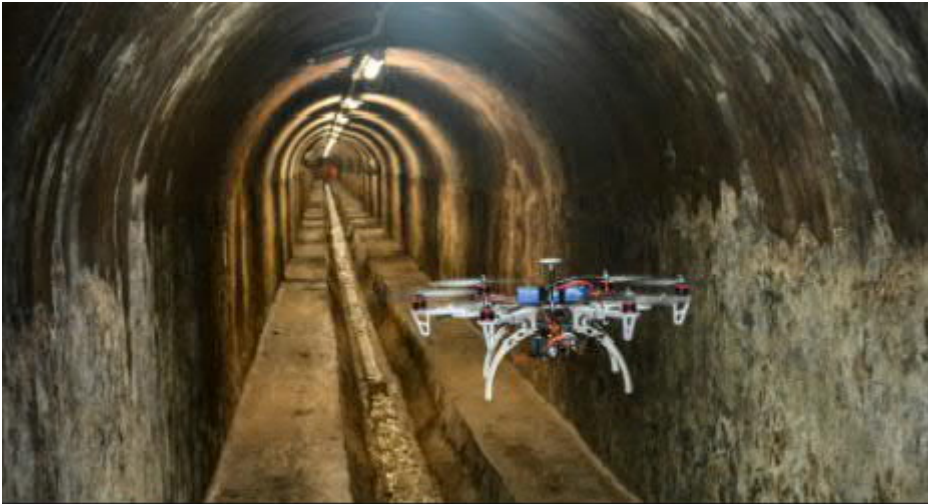
Figure 4.4. Drone with inspection equipment. https://www.thelocal.es/20151207/could-drones-soon-replace-workers-in-barcelonas-sewers
