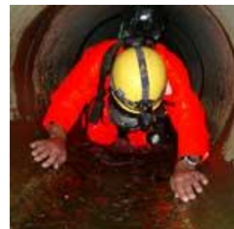
Confined space access requires the correct equipment and training. Picture courtesy of CAS Ltd, UK.
