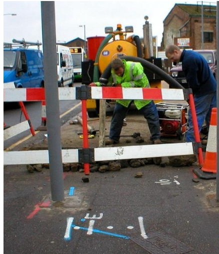
Trail Holing using vacuum excavation techniques. Picture courtesy of U Mole/Infotec.
