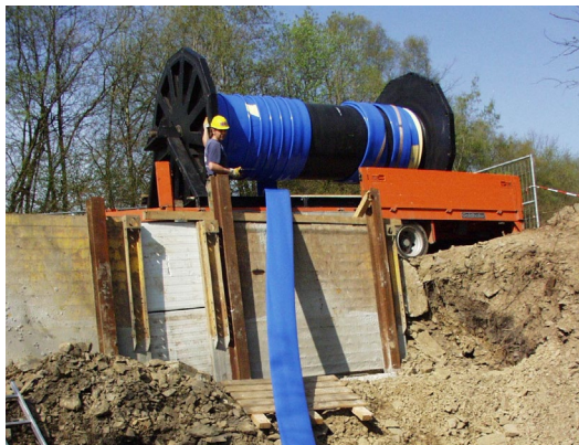
Aramid Fibre Reinforced Polyethylene Lining System
