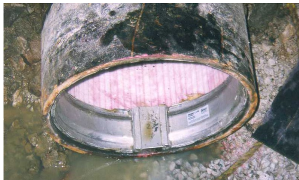
Internal connection seal and backing ring (left) and (right) Seal fitted and expanded.
