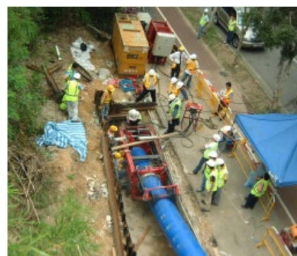
Tension based symmetrical reduction lining systems
