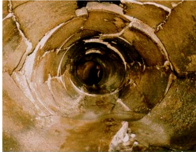
Multiple fractures in a clayware pipe – this is representative of the most severe damage that can be renovated using cured-in-place lining techniques
