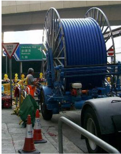
Factory folded Polyethylene Lining System
