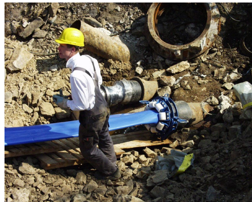
Aramid Fibre Reinforced Polyethylene Lining System
