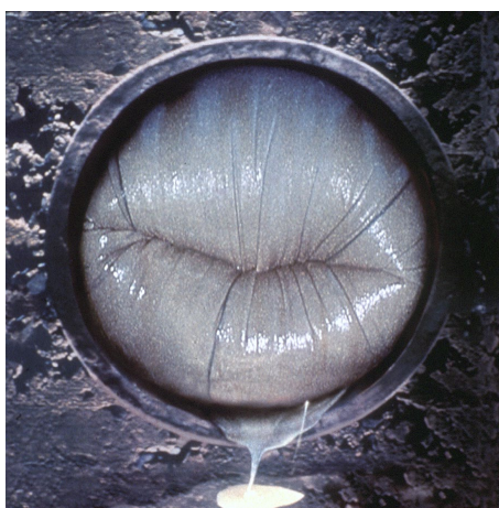
A POLYESTER FELT LNING TUBE (Above) and (below) The INVERSION FACE
