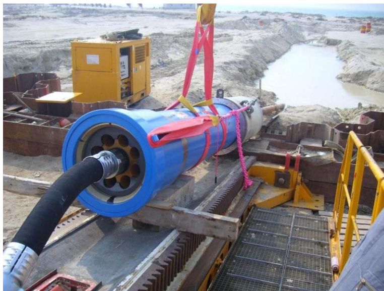
A Ramming Hammer used in an HDD recovery operation. Picture courtesy of Tracto-Technik.
