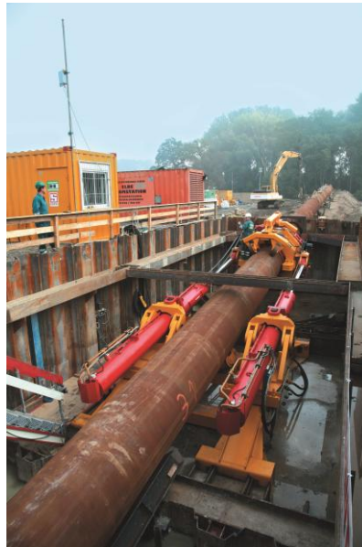
The launch shaft of a DIRECT PIPE installation showing the Pipe Thruster arrangement.
