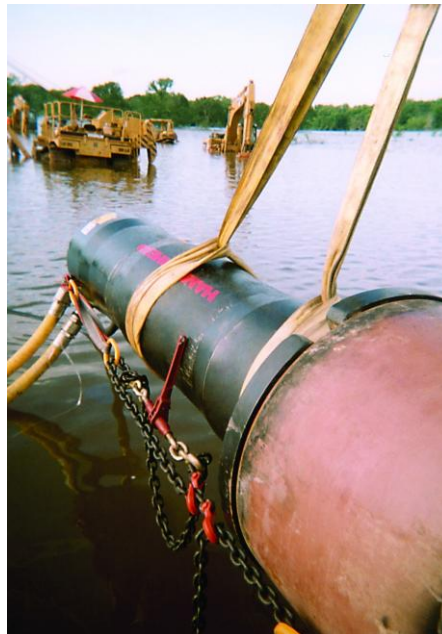
A Ramming Hammer in position to ram a steel casing. Picture courtesy of Earth Tool Corporation.
