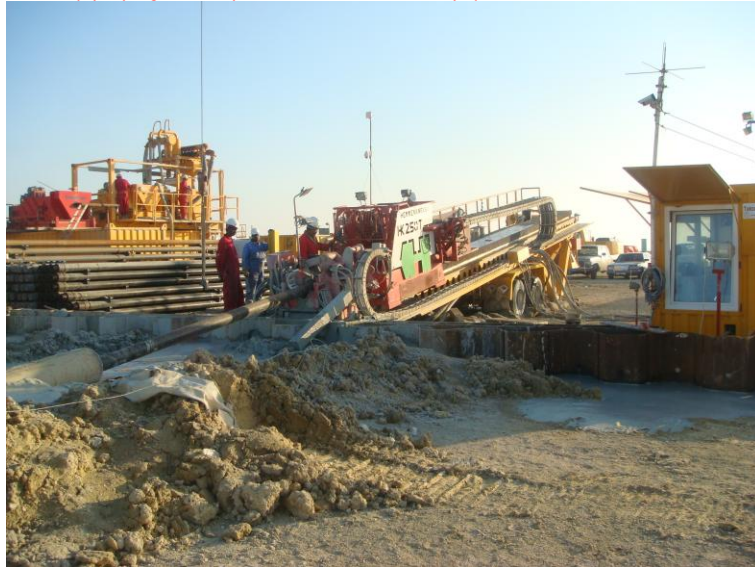
A larger capacity HDD rig. Picture courtesy of Herrenknecht
