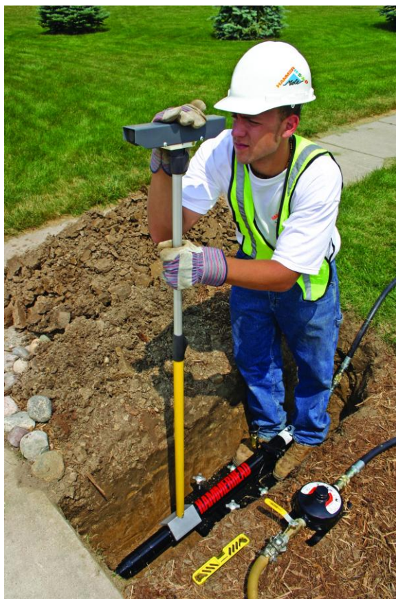
Using a ranging rod to align an impact mole prior to launch. Picture courtesy of HammerHead
