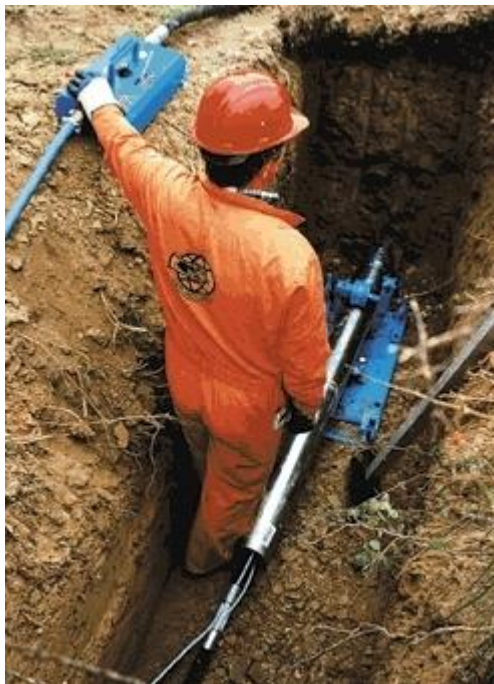
Impact Moling hammer in it's launch pit. Picture courtesy of Tracto-Technik.
