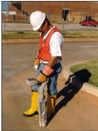
A walkover system tracking an HDD bore.
