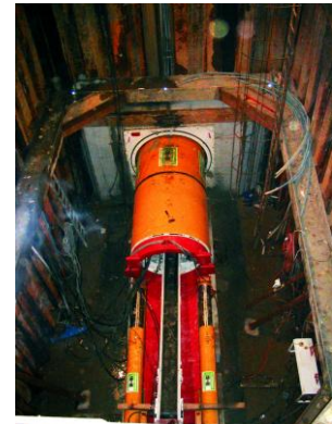
A microtunneller in its launch positioning the shaft. Picture courtesy of Herrenknecht AG
