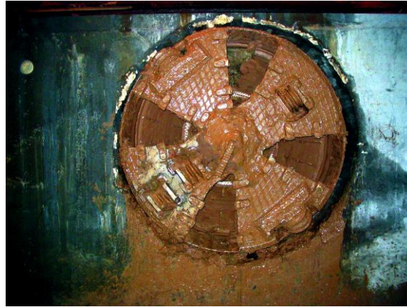
Arrival of a microtunnel cutterhead at a reception shaft. Picture courtesy of Herrenknecht AG
