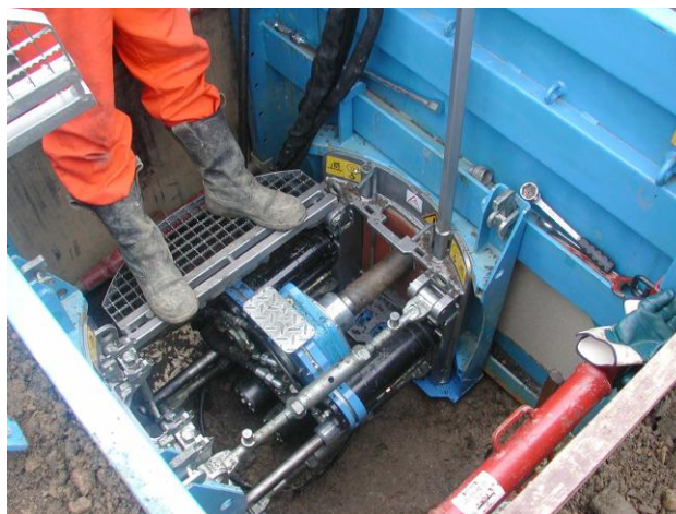
A pit-launched horizontal directional drilling rig. Picture courtesy of Tracto-Technik.
