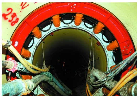
An Interjack Station showing the ring of hydraulic rams. Picture courtesy of Herrenknecht AG
