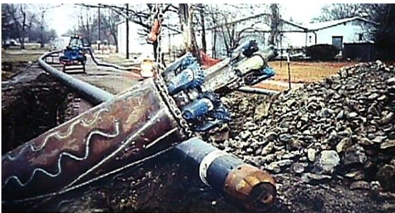
Above: A schematic of the pipe reaming method using an HDD rig as the pulling system. Right: A typical pipe reaming head. Pictures courtesy of Nowak Pipe Reaming.
